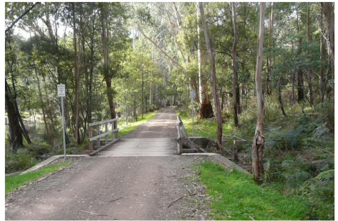
Warburton rail trail bridge on downside of Seville
