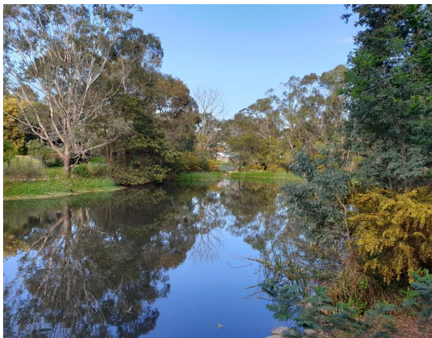
Yanggai Barrage from the viewing platform (JA)
